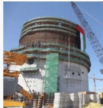
ZheJiang Power Plant Project
