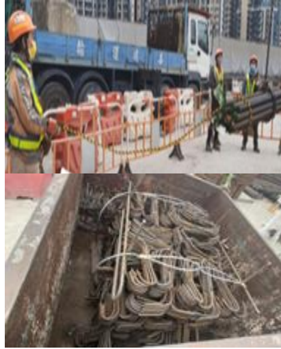
Training and supervising safety lifting operations.
